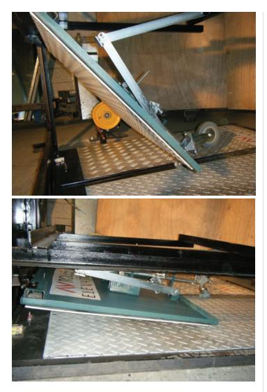
gear mechanism/UCMP of the elevator and operates using an overspeed governor (OSG), rope activation or a solenoid, which, for example, activates an existing anticreeping/UCMP device.
